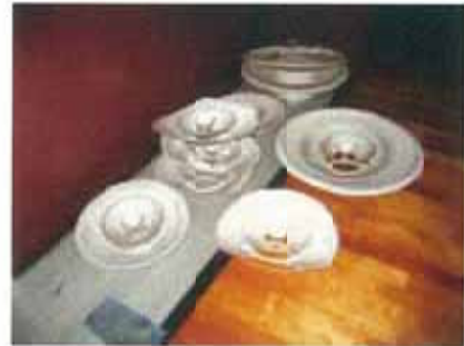
(e)空調噴出し口の脱落
