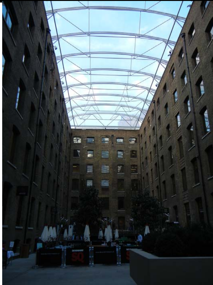
New Street ETFE foil courtyard roof, London
